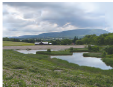
On the cover: The University's Bathgate Dam. Constructed in the early 1990's, the dam has a drainage area of 237 acres and controls peak runoff rates and water quality of stormwater prior to being discharged to the Millbrook Marsh. The back cover photograph is of the Bathgate Dam outflow swale draining into Millbrook Marsh.
