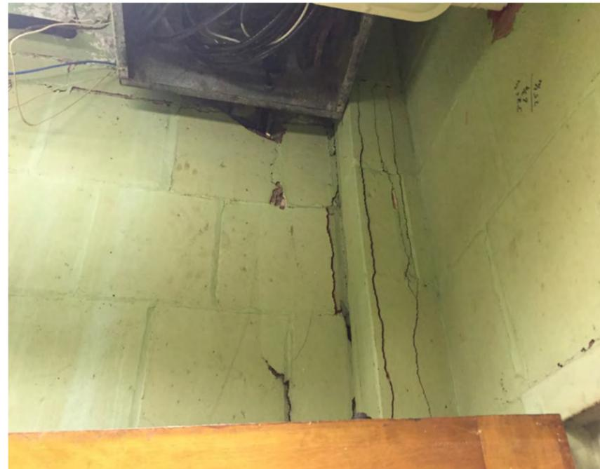
Cracking and Spalling of Sub-basement Storage Room S2 Column Enclosure and Masonry Partition
