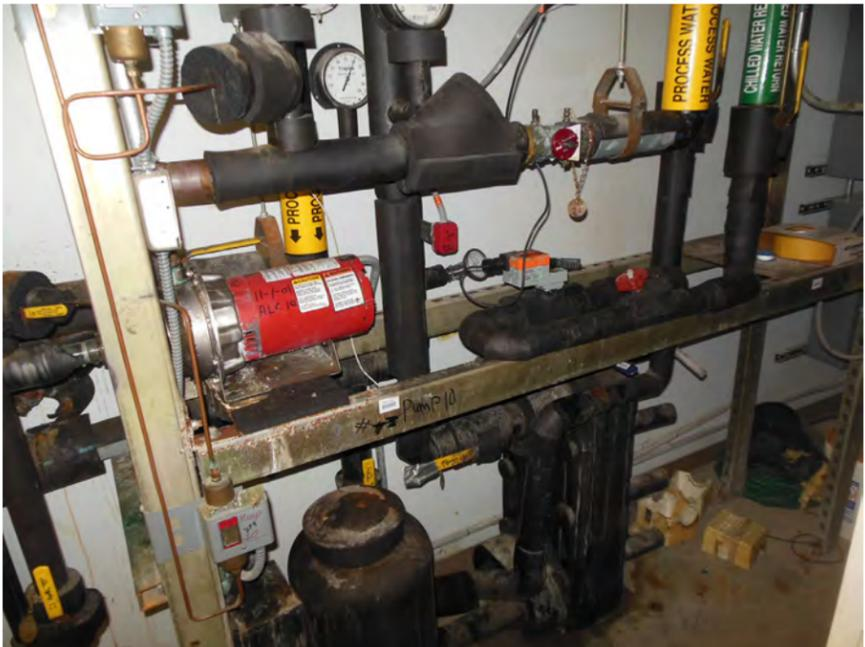
Secondary Chilled Water Pump Loop with Plate and Frame Heat Exchanger
