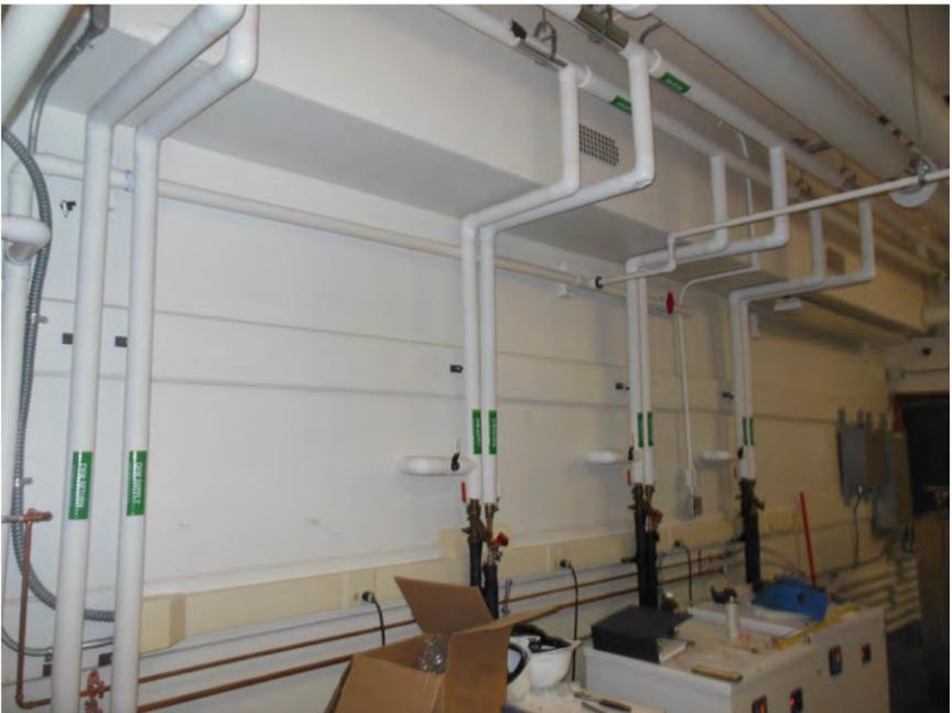
Secondary Chilled Water Pump Loop with Water to Water Chiller
