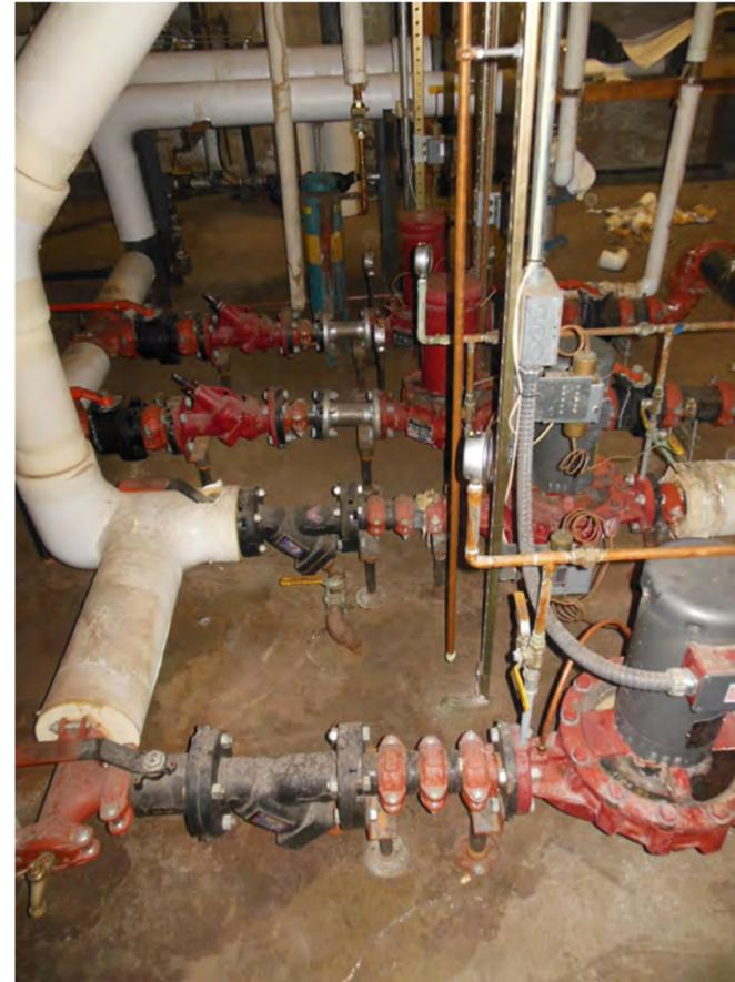
Hot Water Pumping Systems Fed from Steam Heat Exchangers
