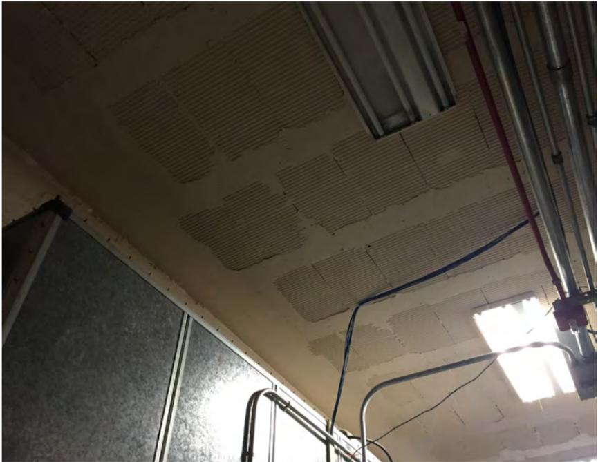
Ribbed Clay Tile Fillers Shown in Between Smooth Concrete Beams
