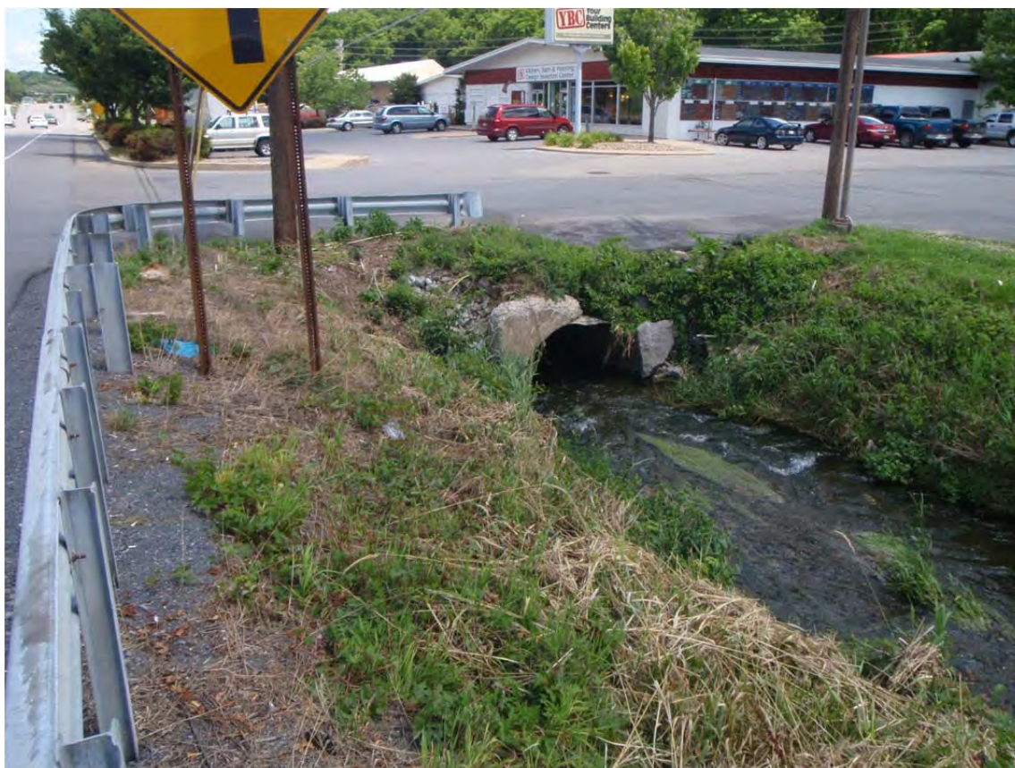
Figure 47. Current Inlet Condition of Clusters' Culvert
