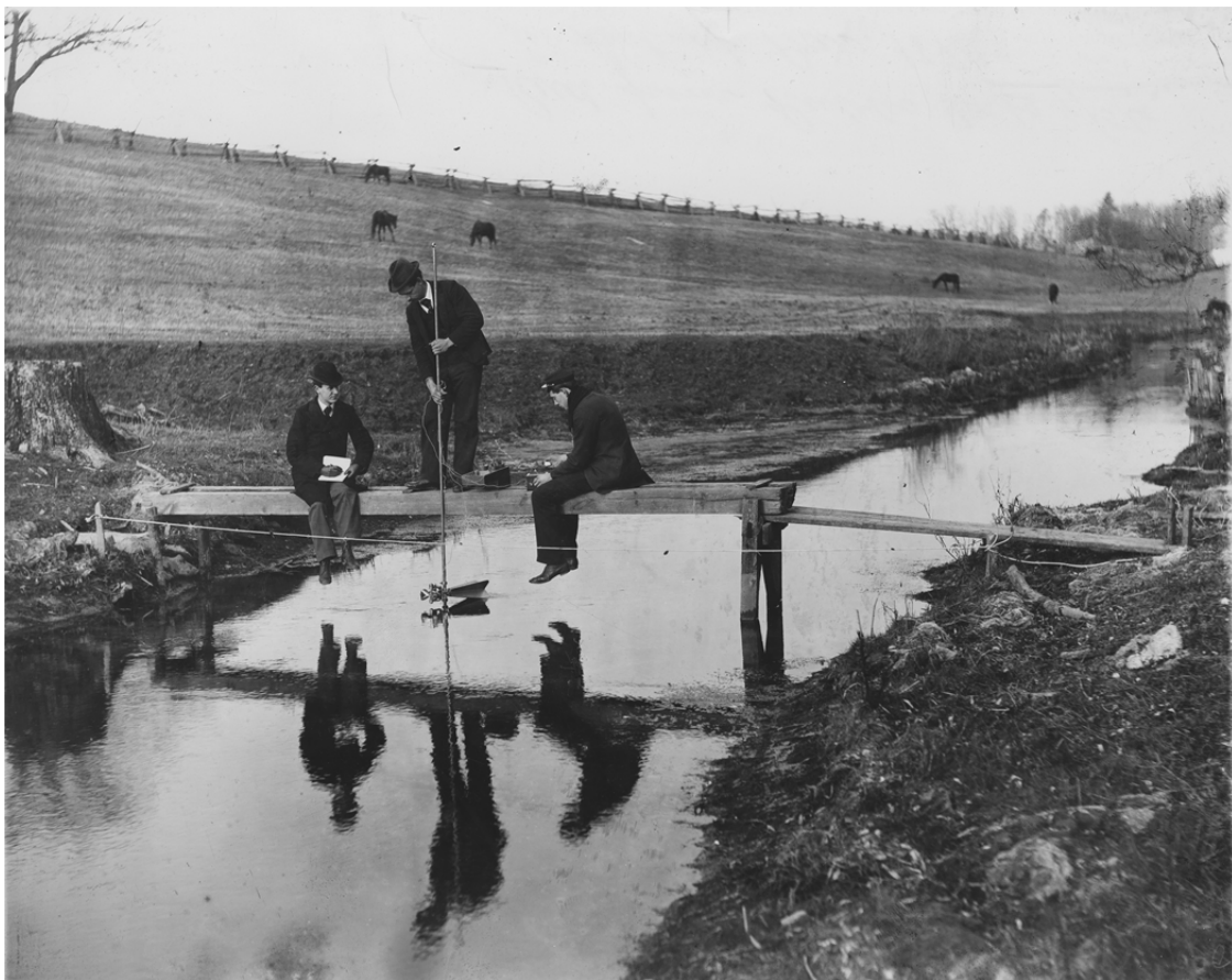
Figure 11. Civil Engineering Students Taking Velocity Measurement on Thompson Run
