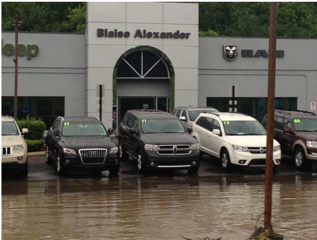
Figure 62. Flooding in Front of Blaise Alexander Auto Showing Ineffective Flow Areas
