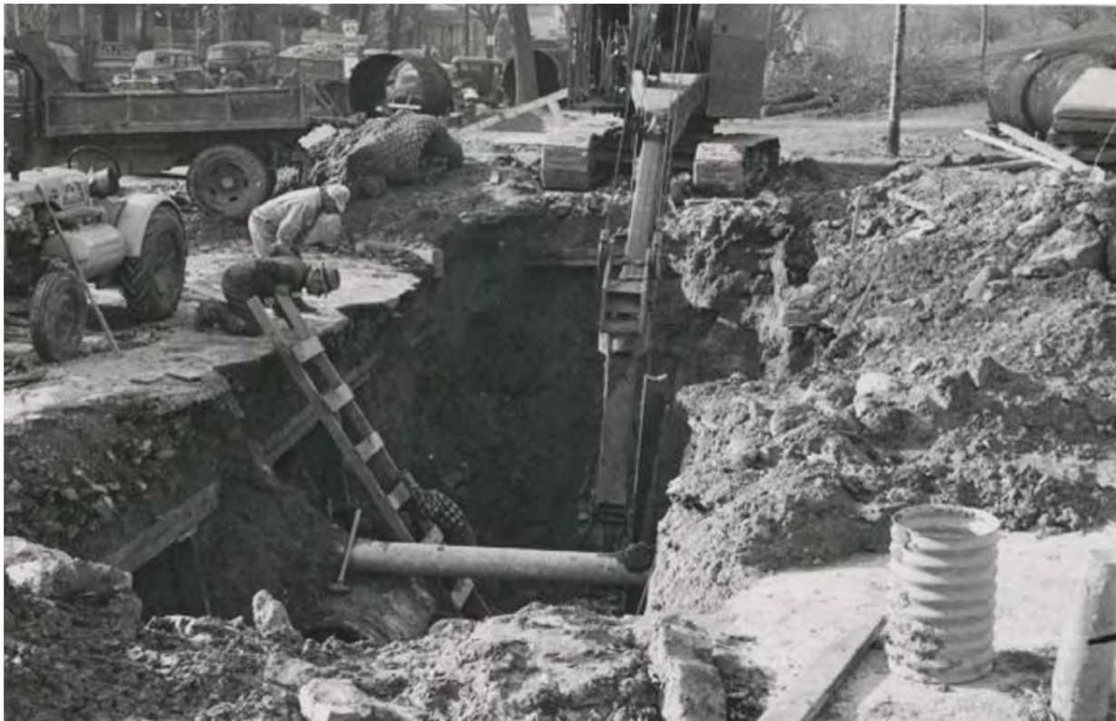
Figure 29. Installation of the 66" University Storm Drain along College Ave in 1948
