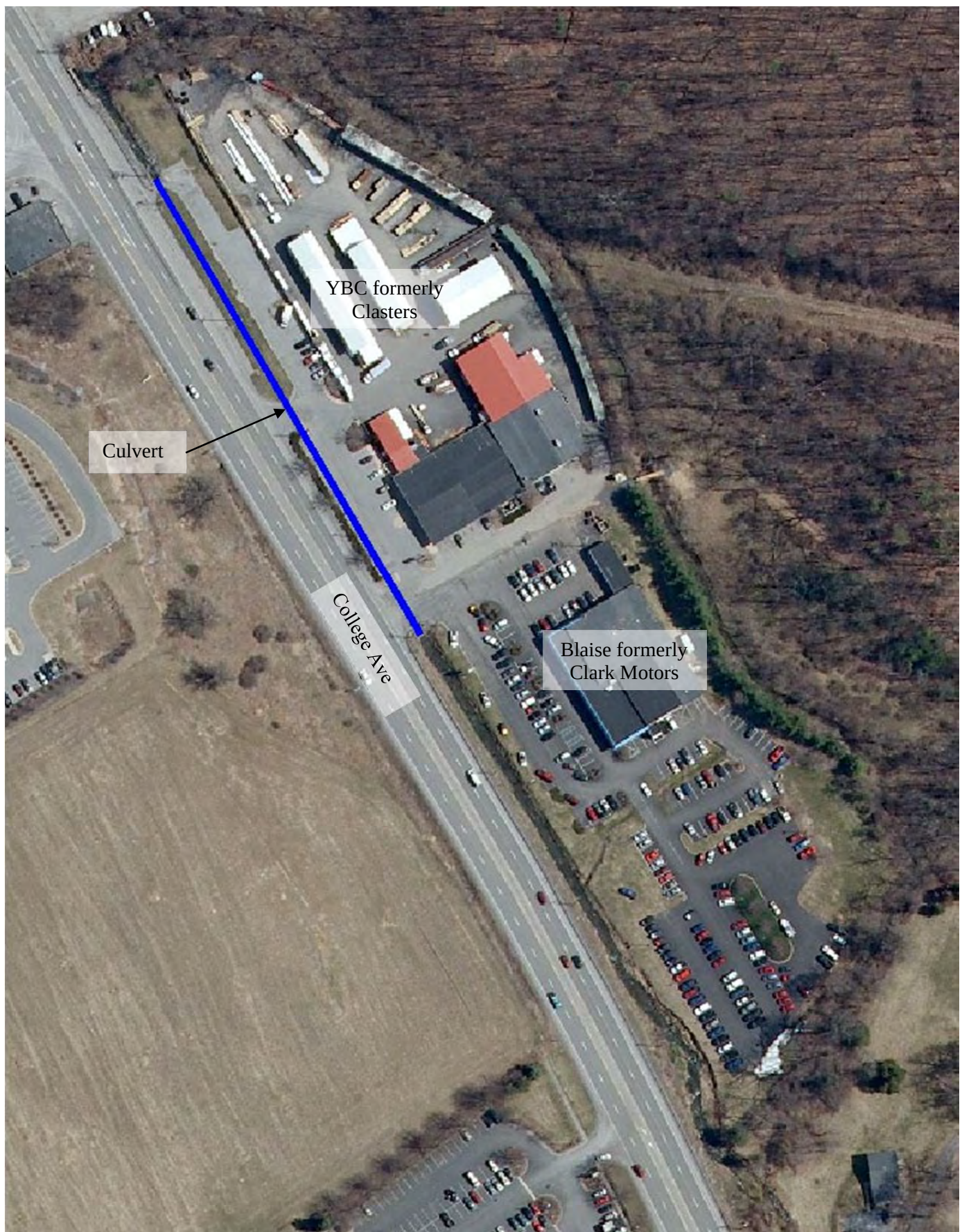
Figure 32. 2010 Orthophotograph with the 1960's Clusters Culvert Shown that Causes Flooding
