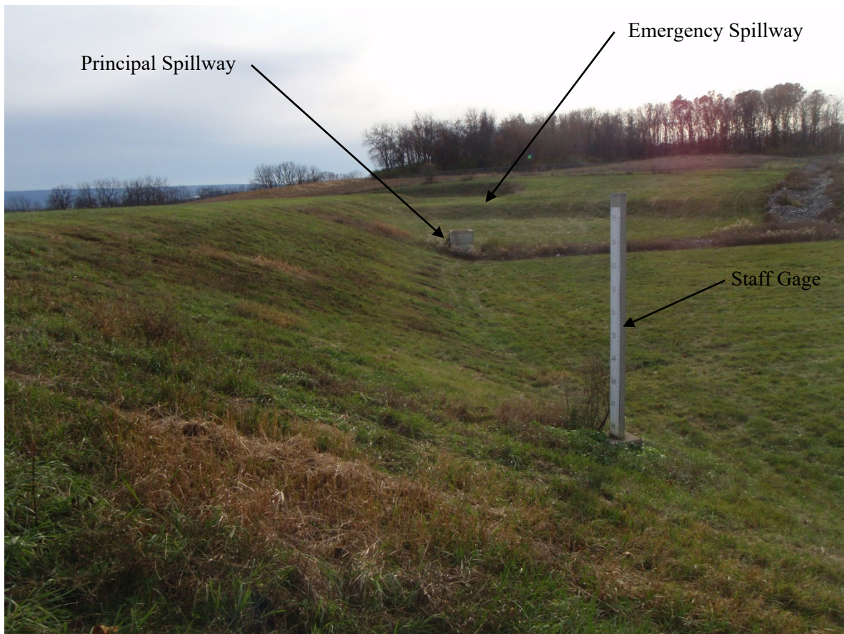
Figure 6. Photograph Showing Staff Gage, Emergency Spillway, and Principal Spillway Looking South
