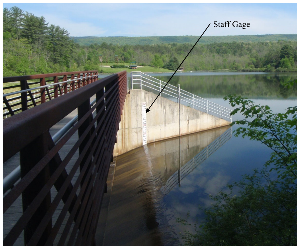
Figure 12. Photograph Showing Staff Gage and Spillway
