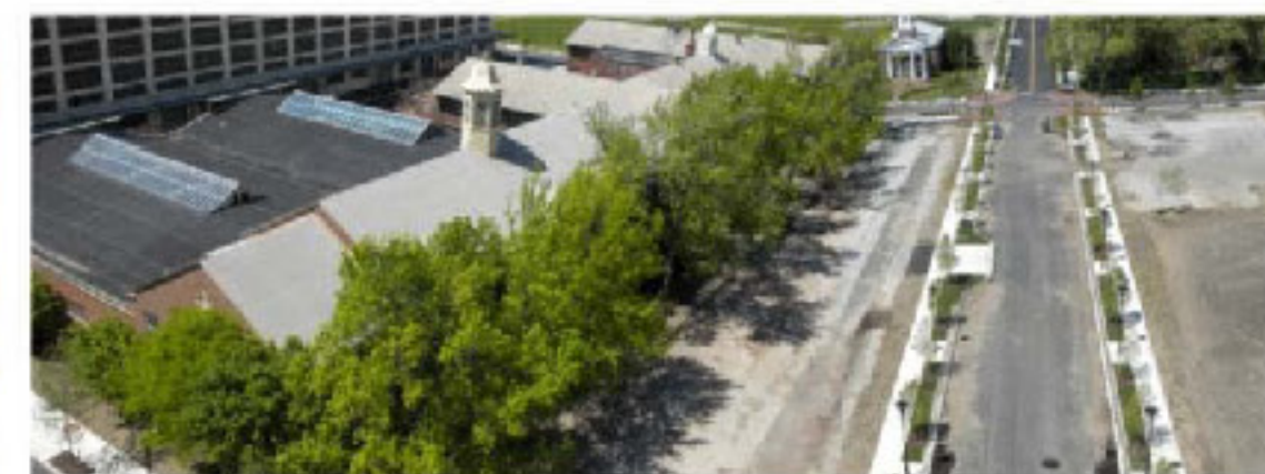
ROOF & PARKING LOT
