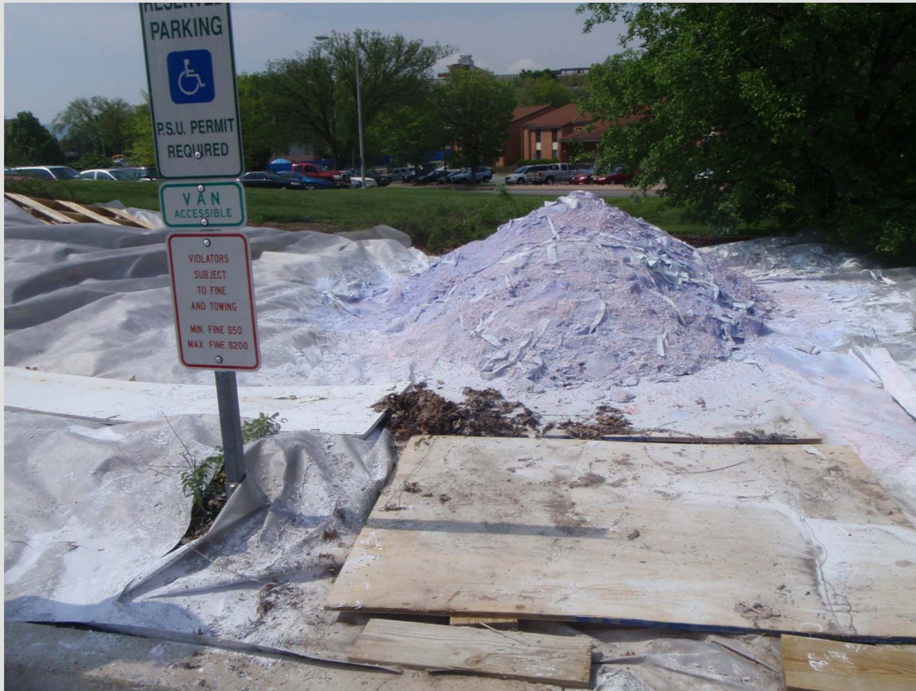
Greenberg Ice Melting over pervious areas using geotextile
