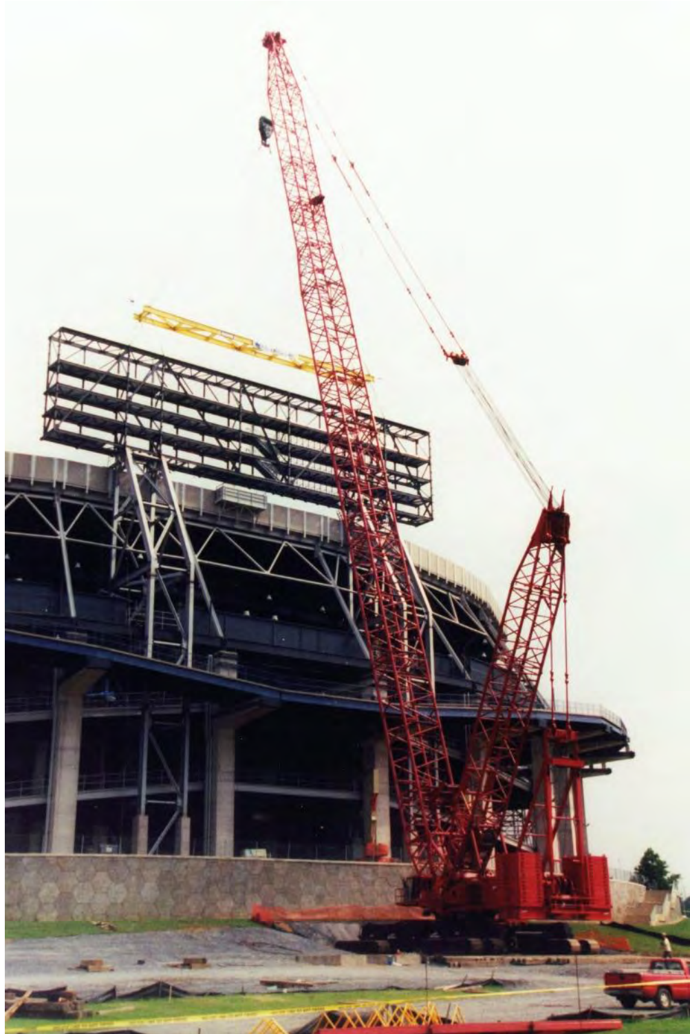
Scoreboard Erection
