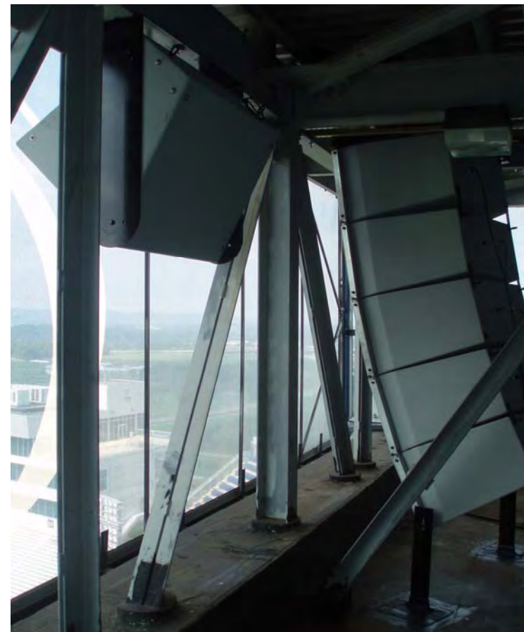
Side Speaker Array & Downfill
