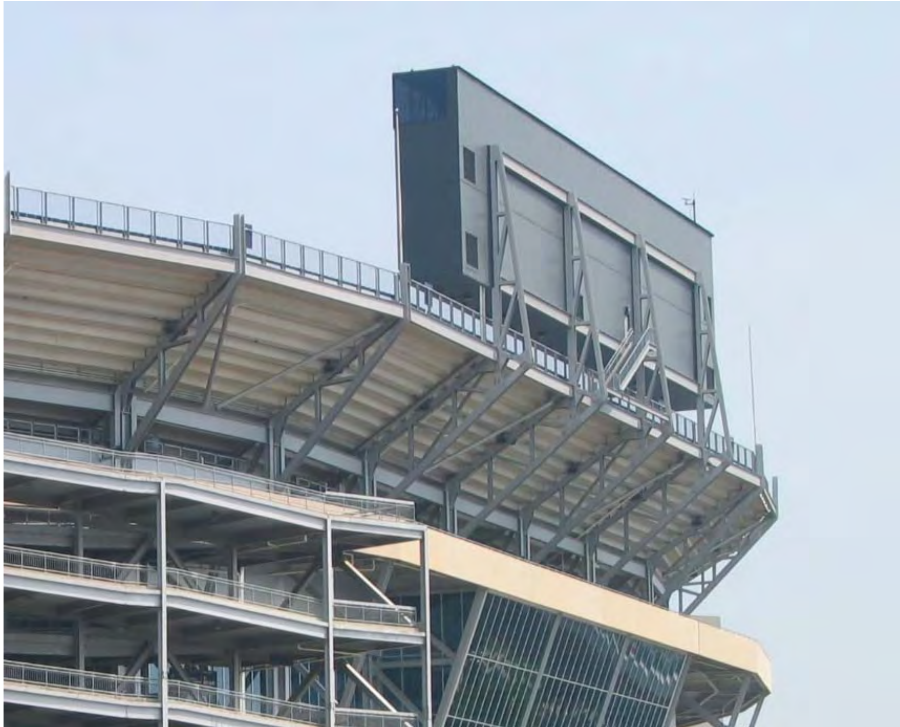
Southwest View of Bleacher Truss Arm Supporting Scoreboard
