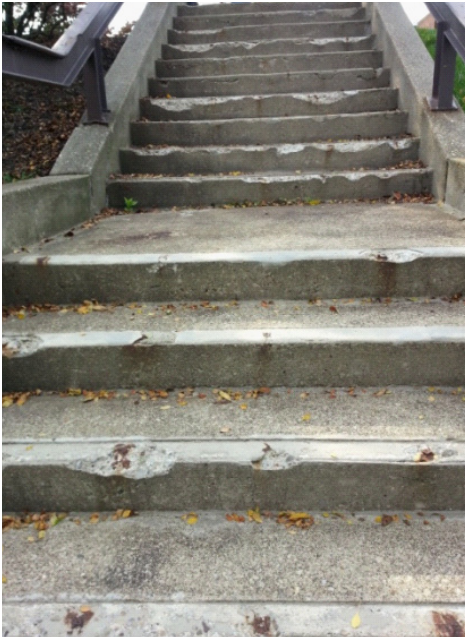
Concrete spalling- Site steps at North Building
