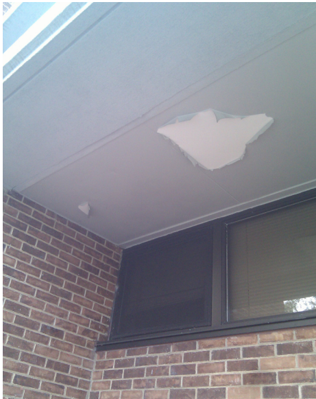
Paint peeling at underside of metal soffits
