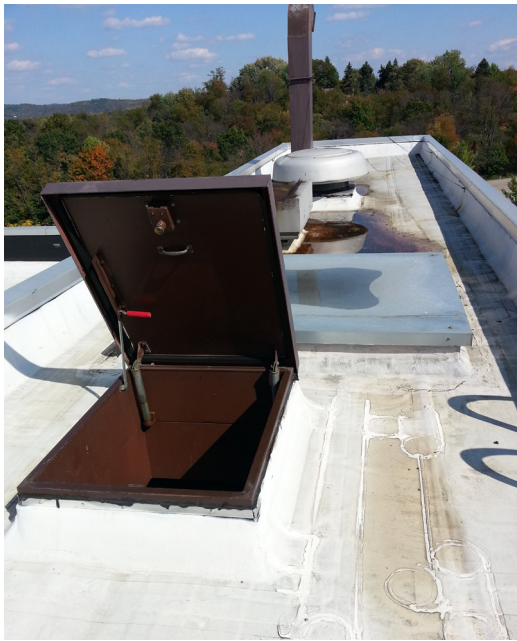
Roof access hatch
